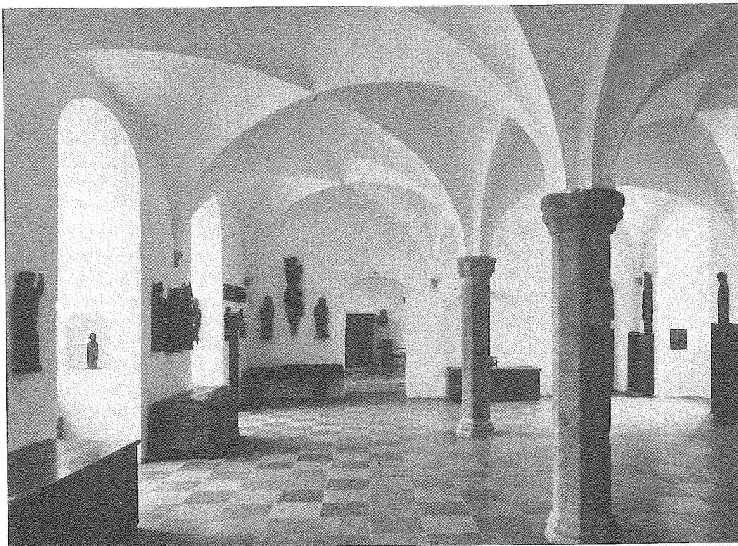
FIG. 2. An exhibition room in the north wing. The vaulted room was reconstructed in 1892 after the discovery of the octagonal granite columns in the town of Kolding. ( Photograph: Ernst Kallese )
